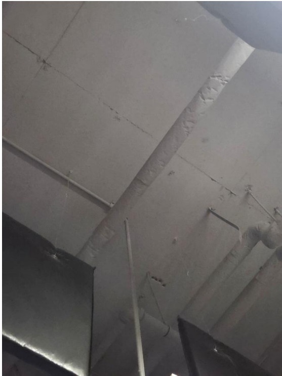
Photo 1: Concrete Slab Framing
