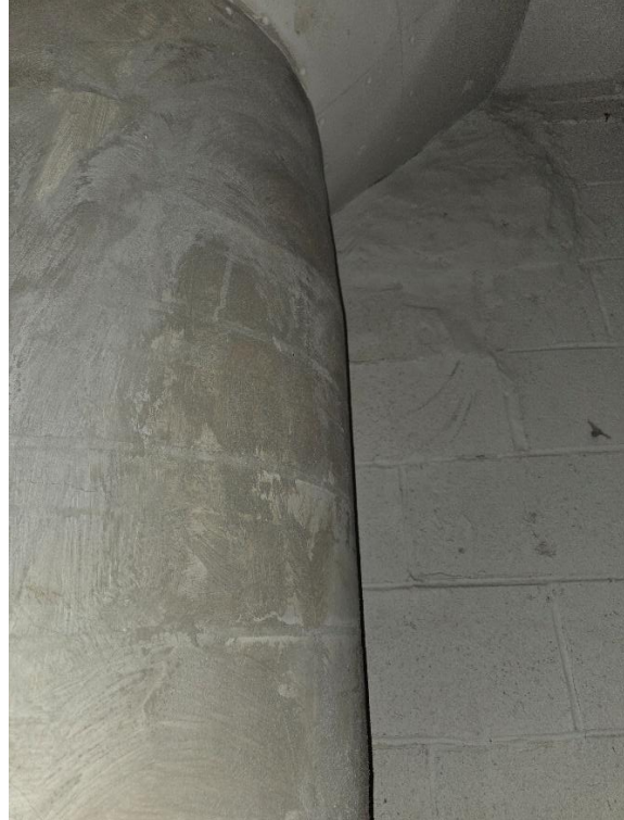
Photo 6: Previously Repaired Column
