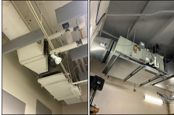
Indoor Carrier Split-System Heat Pump
