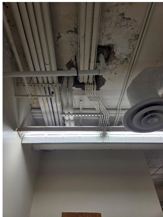
Photo 4: Opening in slab above ceramics room
