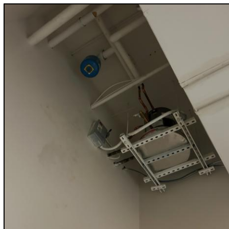
36-Gallon Electric Domestic Hot Water Heater
