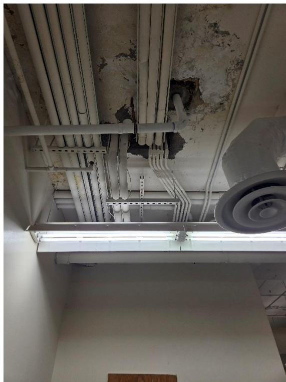
Photo 4: Opening in slab above ceramics room
