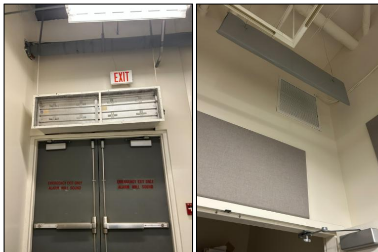
Exhaust Backdraft Damper
