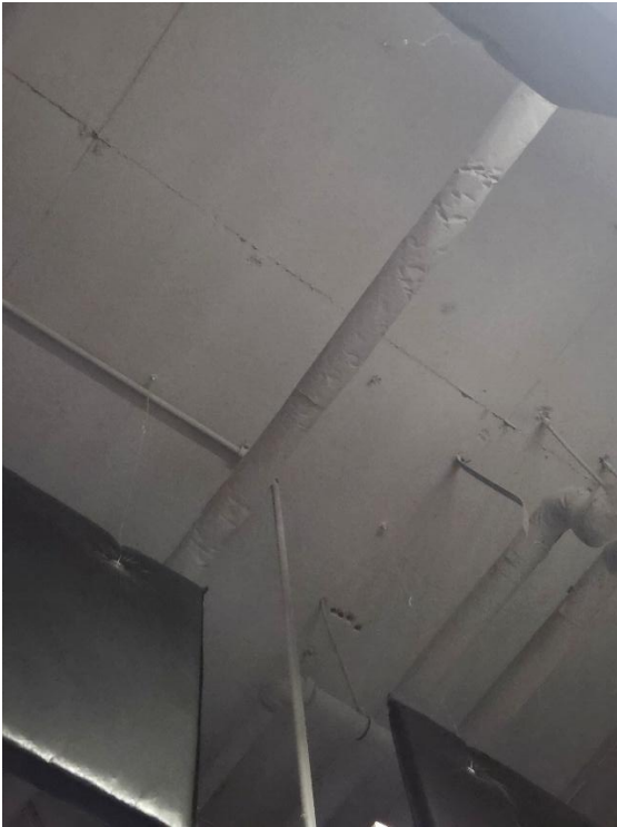
Photo 1: Concrete Slab Framing
