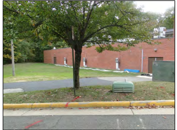
Exterior wall of existing natatorium
