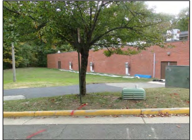
Exterior wall of existing natatorium
