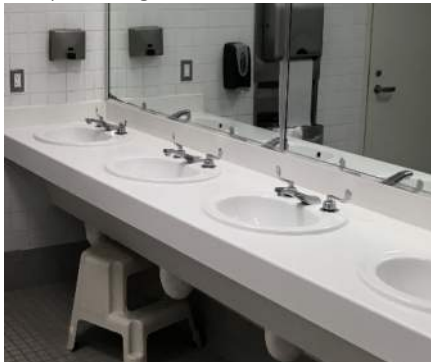
Fig. 31 - Locker room lavatories
