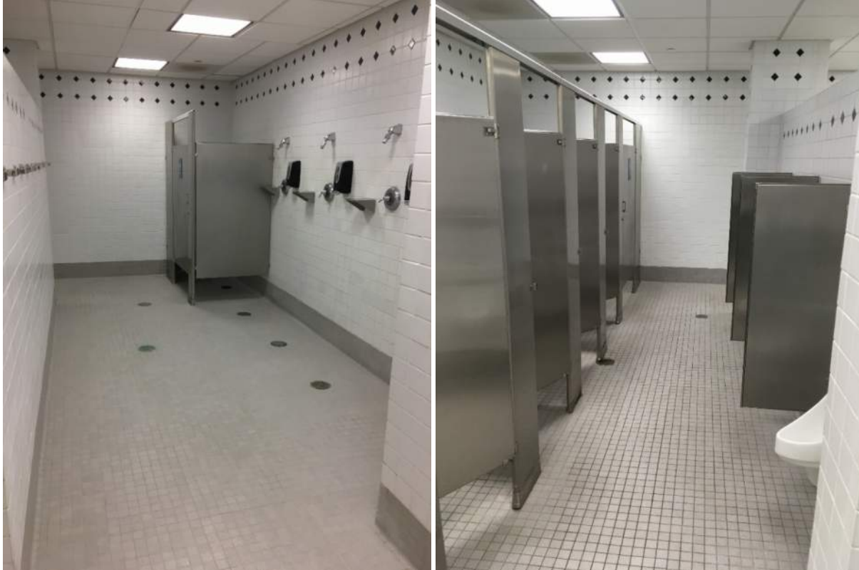
Figs. 18 & 19 - Shower and toilet / urinal area in men's locker room
