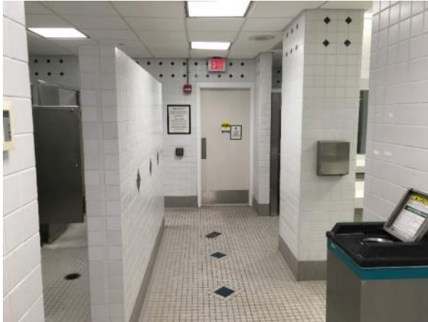
Fig. 14 - ¾ high wall in the women's locker room.
