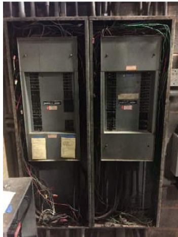
Fig. 36 - Existing panel A
