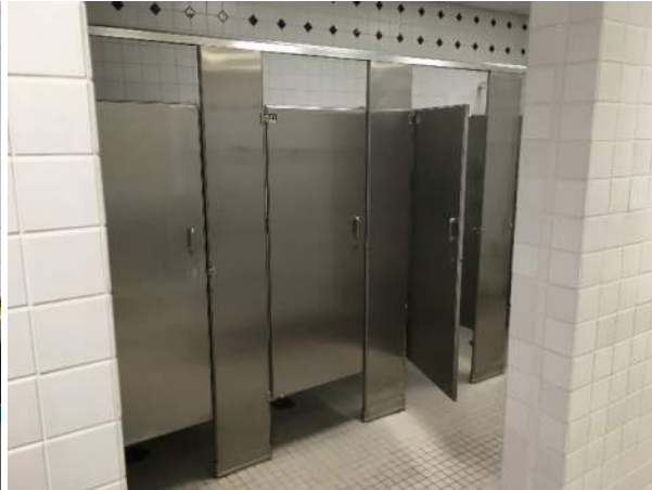
Fig. 15 - Shower partitions at women's locker room
