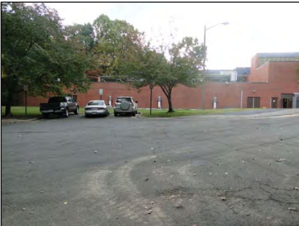
View from parking lot looking at natatorium exterior wall
